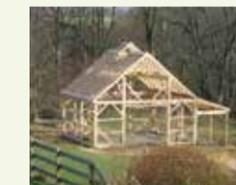
Design features include timber-frame construction done with mortise & tenon joinery and oak peg fasteners. An antique brick foundation (salvaged from local barns) and vertical siding (in traditional red) harken to barns of old. Custom-designed doors that both swing and slide were made using timbers from an old saw mill and are hung on hand-wrought, custom-designed hardware.
