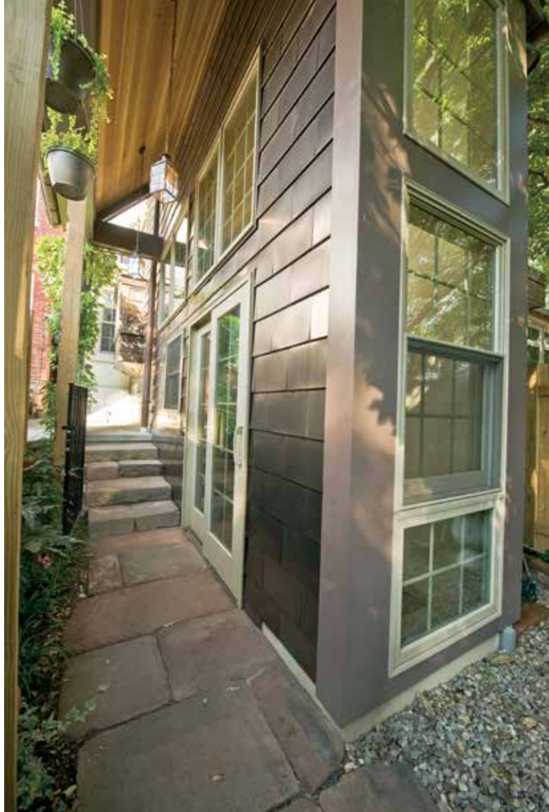
The exterior of the addition is covered with stainless-steel siding, while the underside of the overhang is lined with low-maintenance cedar. Stone that comprises the walkway was reused.
